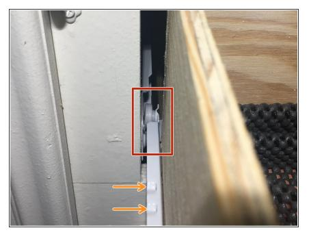
Start by removing the drawer. Pull the drawer out until it stops. You now have 1 or 2 dimples in the track (orange arrows) that stop the drawer from falling out. You have to slightly lift and pull the drawer to continue removing it. When the roller reaches the end-stop (red box), you are ready to pull the drawer up and out of the track.
