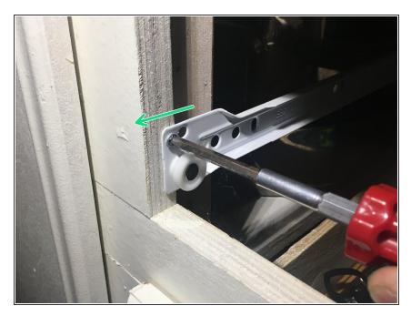
Using your screwdriver, remove the wood screw holding up the track side. Remember: Righty-Tighty, Lefty-Loosy!
