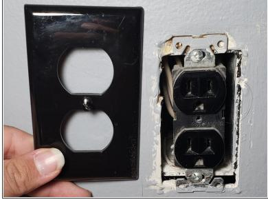
Using a flat-head screwdriver, remove the outer cover plate of the outlet by unscrewing the middle screw.
