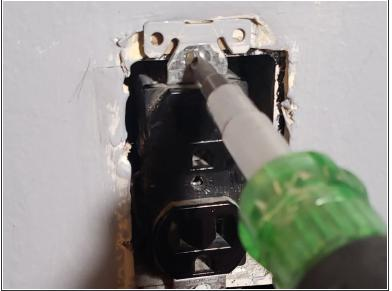
Fully tighten the screws on the top and bottom tabs, positioning the outlet so that it is straight, vertically.
