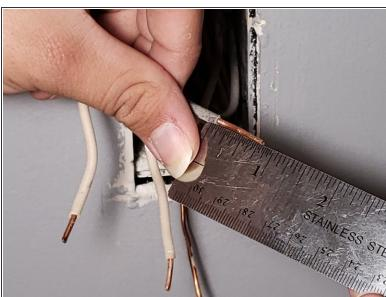
• For each wire, approximately 0.75 inches (2 centimeters) away from the clipped end of the wire, clamp the strippers down on the wire and pull the strippers toward the clipped end of the wire, revealing the bare wire underneath.
