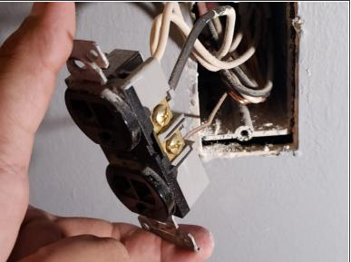
Holding the top and bottom tabs of the outlet, pull the outlet away from the wall, exposing the wires inside the electrical box.
