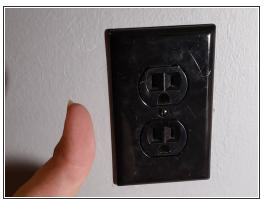
Retrieve the outlet cover plate, and tighten the middle screw to the middle of the outlet.
