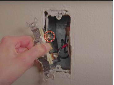
Label the two traveler wires where the up position is held by gold screws of the old switch.
