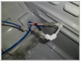
Now you need some plug couplings. Adapter from 6,35 mm (thats 1/4 inch) to 8 mm (thats 5/16 inch), Coupling 6,35 to 6,35 and a piece of hose 6,35. Carefully cut the hose nice and clean with a ahrsp cutter. Now easy click these parts together. Now you have a Bypass for the original Filtermount.:)
