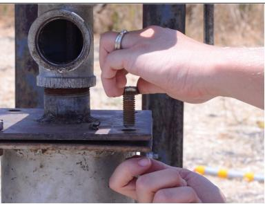
Remove the four nuts and bolts securing the pump riser plate, and store them in a sanitary container such as a bucket.
