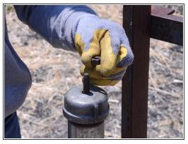
Loosen and remove both the pump rod jam nut and pump rod nut on the top of the slider.
