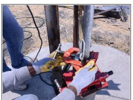
Attach and tighten the elevator clamp to the riser main as close to the bottom as possible.
