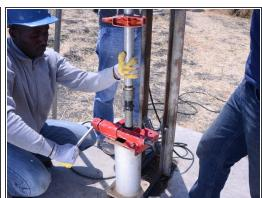
Once the first joint is exposed, tighten the base clamp below the joint.
