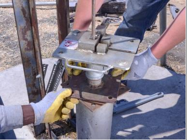
Rotate the pump plate 45 degrees. This will allow for a better grasp when lifting the plate.
