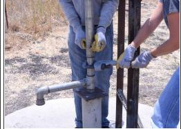
Use a pipe wrench to fully loosen the above grade riser pipe.
