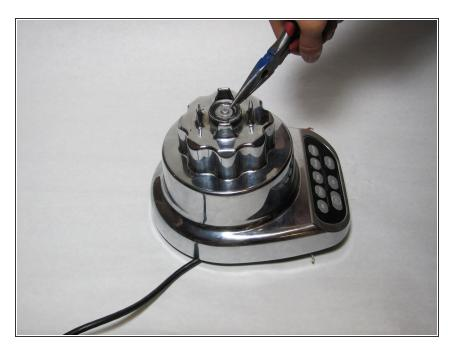
Use the needle nose pliers to turn the coupling clockwise to loosen it.
