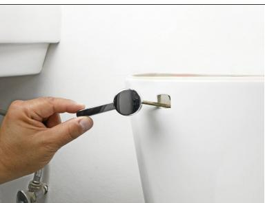
Pull the toilet handle and tank lever forward and out of the toilet tank.
