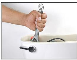
Using an adjustable wrench, turn the locknut on the toilet handle clockwise until it loosens.
