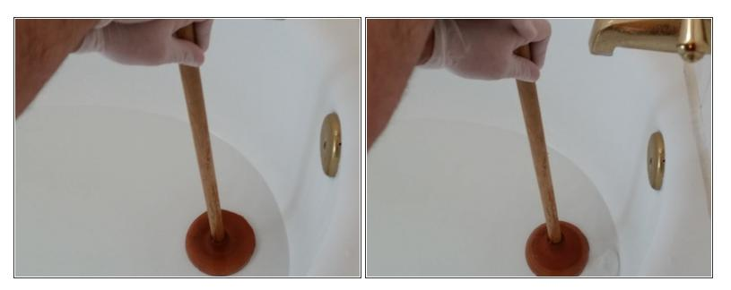
Without breaking the seal of the plunger on the drain, push the plunger sharply down and up a few times.
